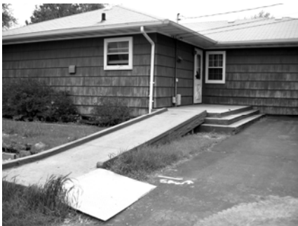
Ramp at Attewell home built by Logan's foundation
